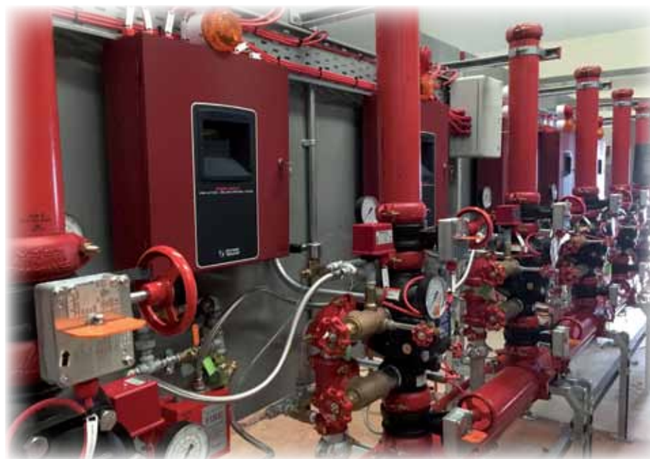
Pre Action Valve and Control Panel Skid sets
