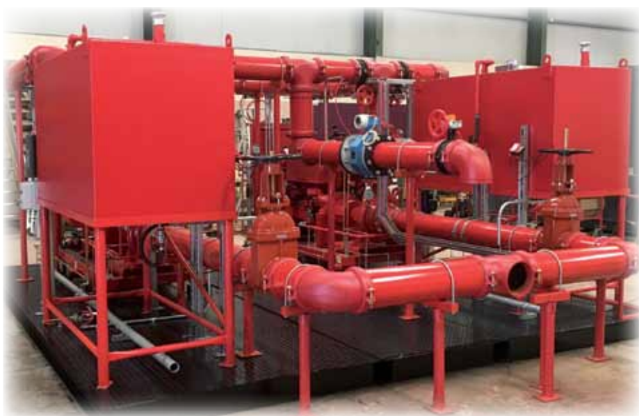
Fire Protection System (Pump room skid) shipped to Bahrain (FM Approved)
