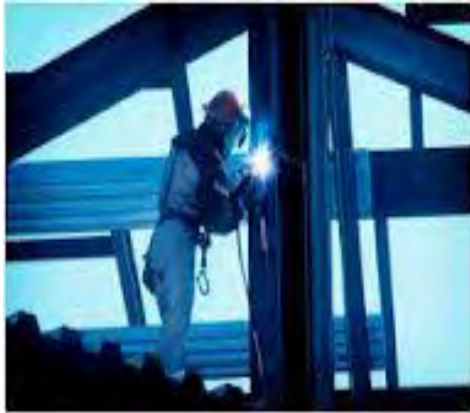
Electric Arc Welding
