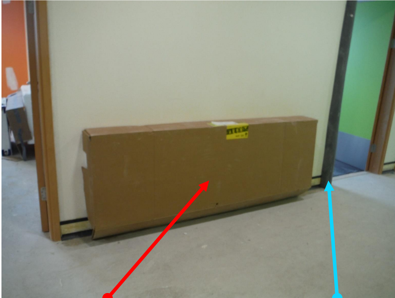
Cardboard protecting wall heater
