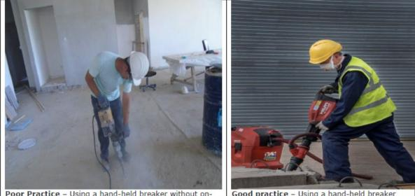
Poor Practice – Using a hand-held breaker without ontool extraction (DLI, CY)
