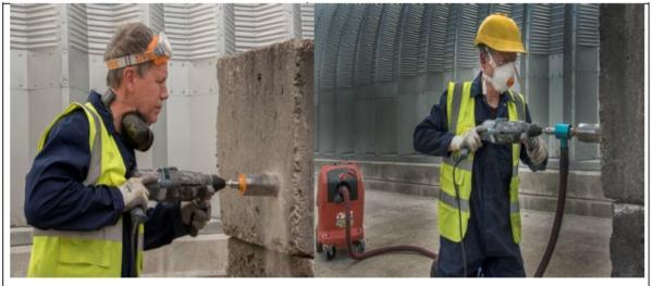
Poor Practice – Using hand-held corer with no extraction or RPE (HSE, GB)
