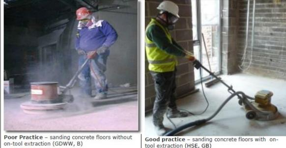
Good practice - sanding concrete floors with ontool extraction (HSE, GB)
