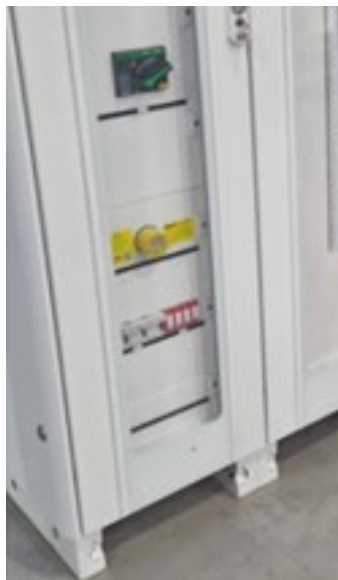
Figure 4 - Front and Rear Plinth Covers Removed for Movement
