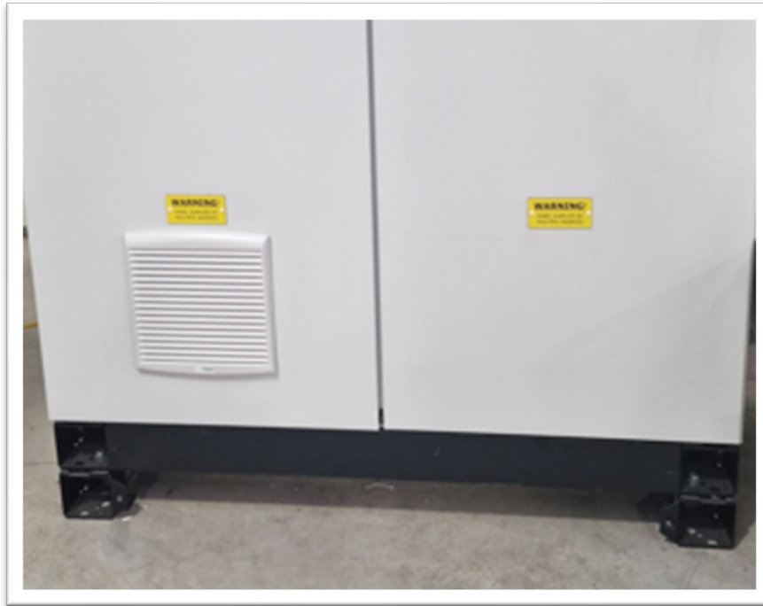
Figure 5 - Front and Rear Plinth Covers Reinstated
