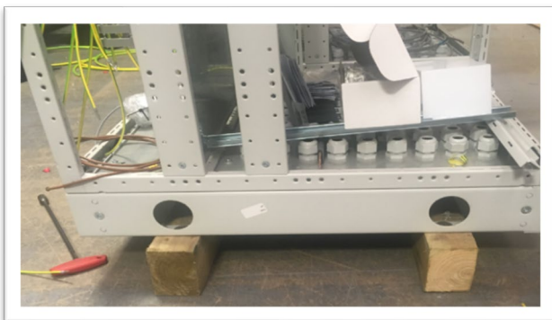
Figure 12 - Access Points for Lifting (with removable covers)
