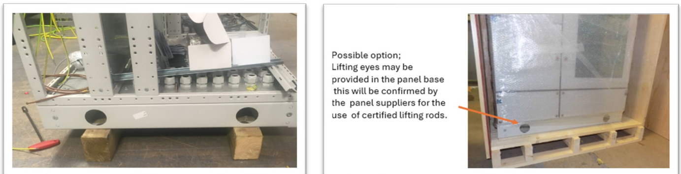
Figure 12 - Access Points for Lifting (with removable covers)
