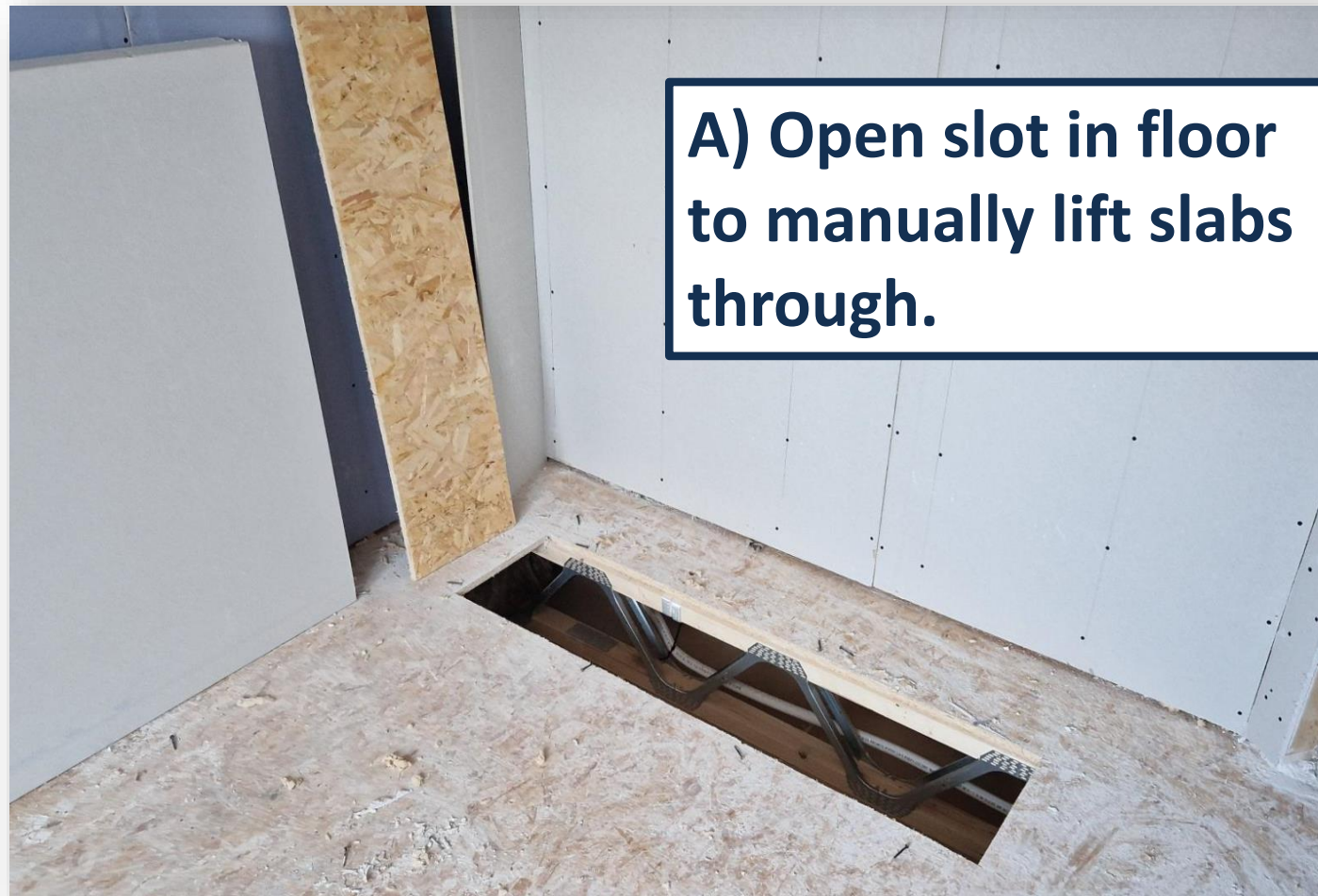
loading out on Ground Floor Concrete slab during timber frame install – No issues
