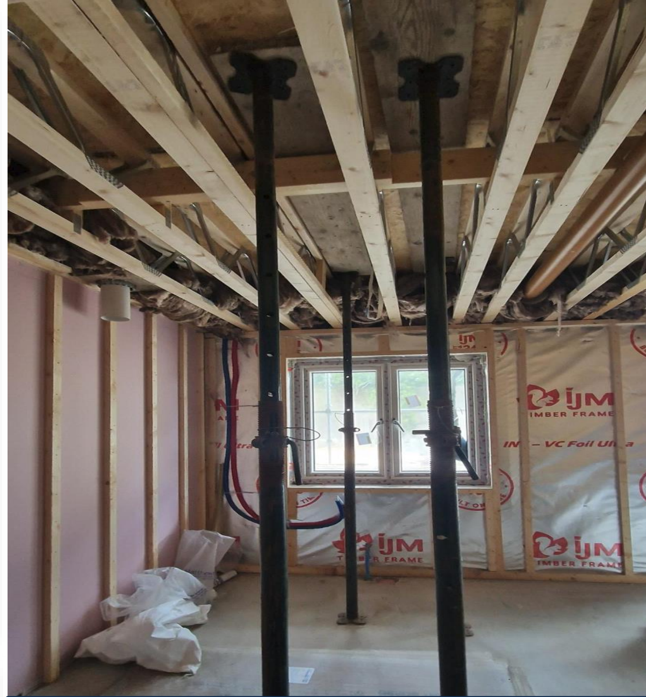
B) Prop flooring and load out slabs using crane during timber frame install.
