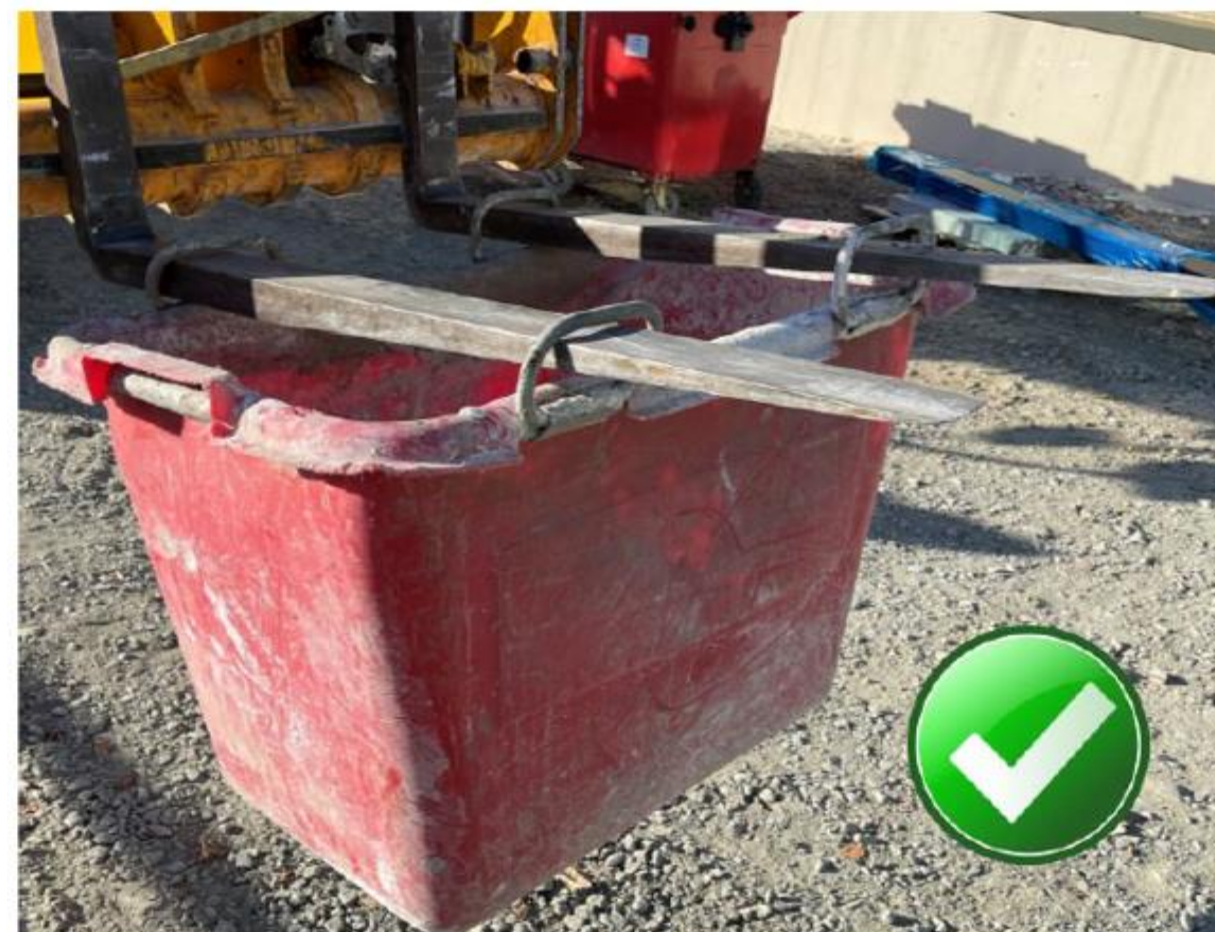
Image E. Correct lift– forks through Mortar Tub lifting square-eyes.
