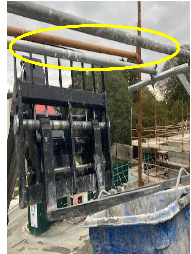
Scaffolding ledger obstructs lift when mortar tube is lifted by lifting eyes, There is then a tendency to lift mortar tub by pinching sides of bin.
