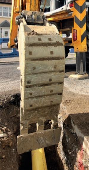
Mechanical excavators pose the highest risk and “should not be used within 500 mm of a gas distribution pipe.”
