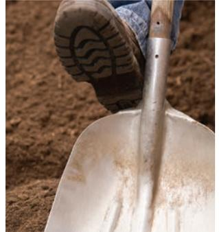
Hand digging using shovels and spades presents the lowest risk of damaging a gas pipe.
