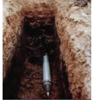
**Moling/Directional Drilling** – installing mains/ services where a 'moling' machine drills from one location to another pulling the pipe behind it using "no-dig" technology.
