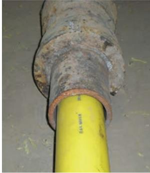
**Insertion** – utilising existing metal gas mains / services as a carrier for new PE pipes. Inserted PE may be a close or loose fit. The carrier pipe is broken out at connection points, i.e. at pipe joints or where a gas service pipe is connected.
