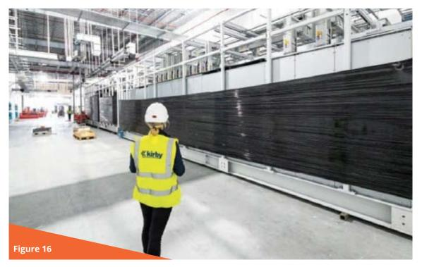
Kirby Group Engineering offsite fabricated Electrical Switchgear module *July 2020.*
