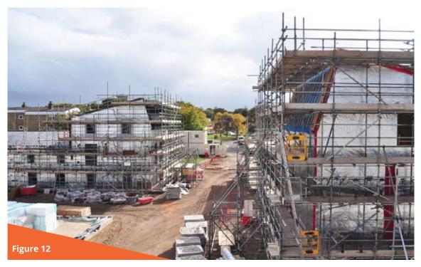
**Cygnum** onsite erection of offsite fabricated components *11th November 2020.*
