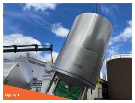
Brodeen Fabrications, Tipperary modular Vessel fabricated offsite for installation in Tipperary Co-operative 21st June 2021.
